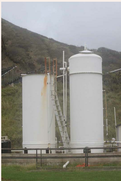
Figure 1 Pilot test plant installed at East Honolulu Wastewater Treatment Plant's (EHWWTP) premises in Honolulu. The tower on the right is anaerobic packed bed (AnPB) reactor operated in upflow mode and the column to the left is a trickling filter.
