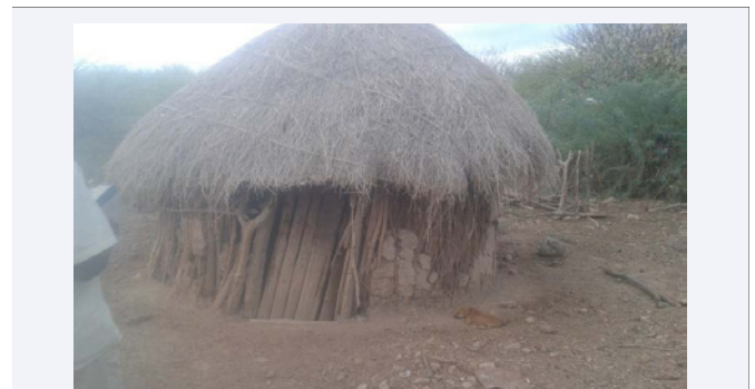
Figure 3 Mud-walled, grass-thatched house (Photo by Nzau 2016).
