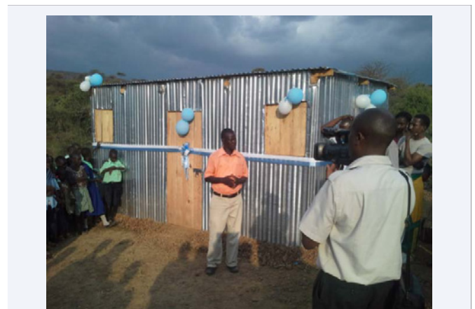
Figure 4 The new structure of the improved house (Photo by Nzau 2016).
