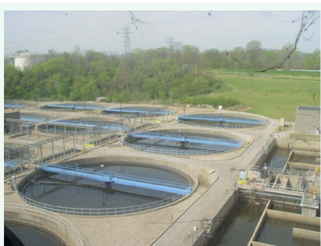
Figure 1 Metropolitan Municipal Wastewater Treatment Plant, Louisville, KY.
