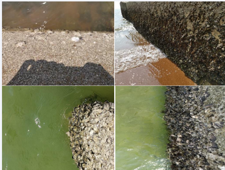
Figure 5 The inside view of various outfalls at Port Dickson's beaches.
