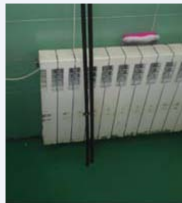
Figure 4 After removal of two rebar.
